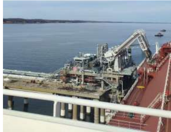
Figure 1. Loading arm and manifold installation activities
