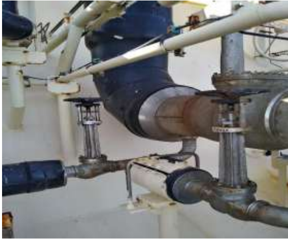
Figure 2. Loading arm and manifold installation activities
