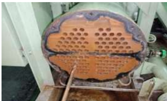
Figure 1. Clogged Condenser
