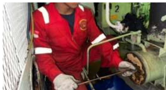
Figure 2. Condenser Cleaning Process
